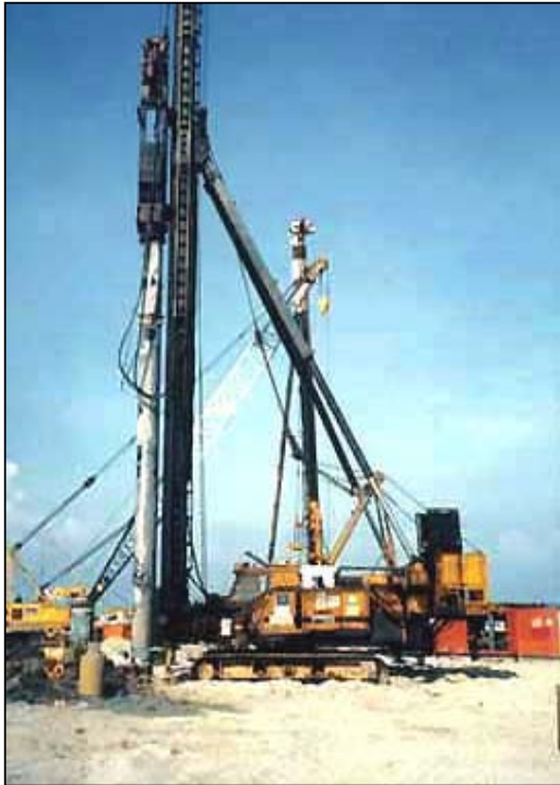
Figure 1A: Actual Pile Driving System
