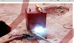
Joint-welded YJACK to starter pile section(s) (joint-welding follow contractor SOP)
