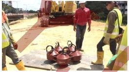
Ready a flat working platform at site by contractor (locate YJACK on the flat plywood/steel platform)
