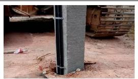
Continue driving the pile with YJACK until pile set (pile driving criteria follow contractor SOP)
