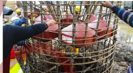
Continue cabling when lowering down the rebar cage (fasten with cable ties along the rebar cage)
