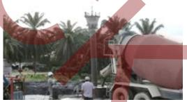
Lower down the tremie pipe and concreting (slowly and carefully follow contractor SOP)
