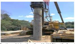
Continue driving the pile with YJACK until pile set (pile driving criteria follow contractor SOP)
