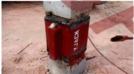
Joint-welded extension pile section(s) to YJACK (joint-welding follow contractor SOP)
