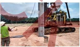
Connect hoses and telltales along the pile body (use poly pipes as protections, if necessary)
