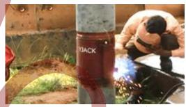
Joint-welded extension pile section(s) to YJACK (joint-welding follow contractor SOP)
