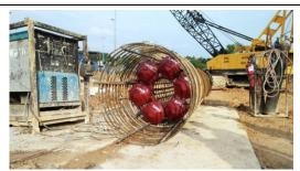
Lower the connected YJACK on to ground (horizontally to connect hoses and telltales)
