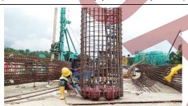
Connect YJACK perpendicular to the rebar cage (vertically by welding YJACK on rebar cage)
