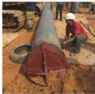
End Bearing SC600Ø
