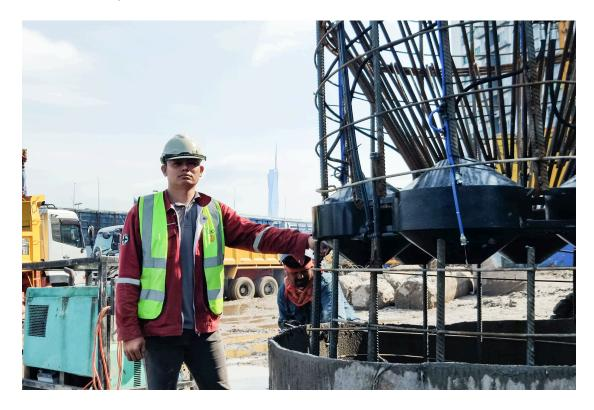
One of the standout features of the YJACK BDSLT is the reduction in machinery required during the pre-installation phase. Traditional pile load tests often necessitate the use of extensive equipment to set up the test apparatus, including cranes, concrete blocks, and other heavy machinery. This not only increases the complexity of the setup but also poses safety risks associated with operating large machinery on-site.
